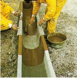
*Lastois canalones is a product based on bicomponent resins and consistencies gel type, with great adhesion and elasticity ideal for the waterproofing of gutters.*
