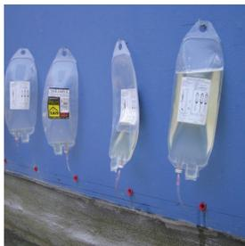
*Teias Capi-C is a system that consists of injectors so as to protect against rising dampness. It is based on special resins with great damp-proof and waterproofing power. Its great fluidity ensures excellent penetration into the pores until reaching the point of saturation.*
