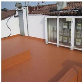
*Lastois fibro is a waterproofing based on styrene acrylic resin, presenting thixotropic consistency and incorporating special fibers. Specially developed for getting durable flexible waterproof membranes.*
