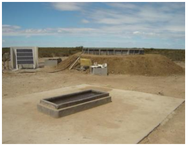
PV for pumping water in C. de Patagones
