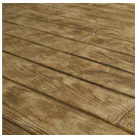
**Imade** is a paint based on synthetic resins that apply on mineral substrates such as concrete and mortars, provides a look similar to wood.
