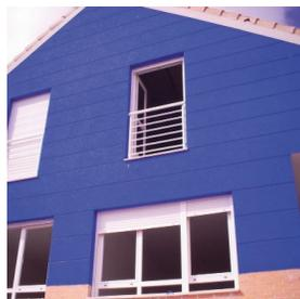
*Teais Homocolor is a resin with high adherence and excellent resistance to weather that improves and enhance the covering colours based on monolayer mortars.*
