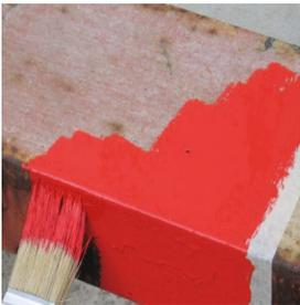
*Pintox is an enamel based on resins with special additives which provides to it anticorrosive properties.*
