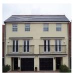
**Repois R** consists of a cement based external through coloured render. It is formed by a mortar that is freshly applied and allowed to dry partially. A special trowel is then used so as to obtain a decorative scratched finish.
