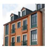
**Relais** consists of an acrylic texture coating system that is trowel-applied in interiors and exteriors. It is composed of vinyl resins and selectively graded agaregates and additives.
