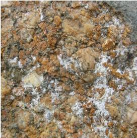
*Limsal is a liquid product specially designed for cleaning superficial salts in several supports in construction. LIMSAL forms a thin coat that softens and attack salts removing them.*
